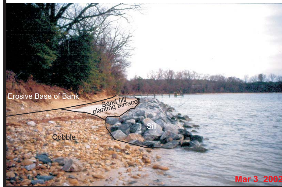
Figure 1-6 . Photos of Window 8 showing the elements of the sill project. These photos were taken before the marsh grass was planted.
